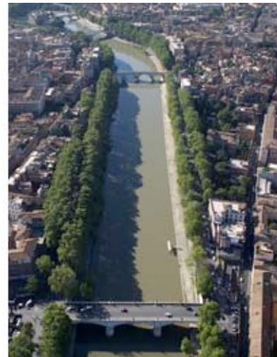
Fig. 7b: Aerial View of Piazza Tevere. Alex S. MacLean.
